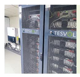
"The size and orientation of the PV installation means we need high charging and discharging power for the building, which the TESVOLT storage system provides with an output of 120 kilowatt. The storage system we installed significantly increases the self-consumption of this innovative, state-of-the-art living concept."
